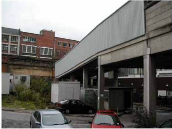
View of Overhead Connection
