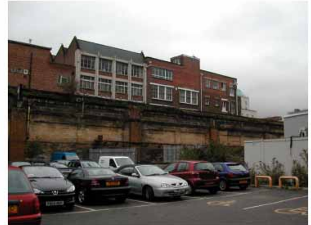
View towards Bold Street
