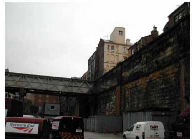
View of Heathfield connection to Street
