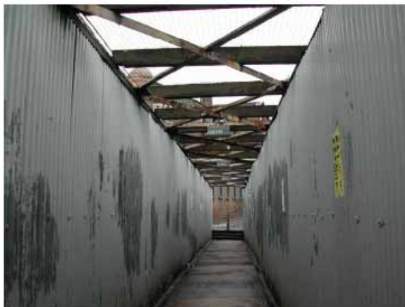
Heathfield Pedestrian Crossing looking towards Copper
