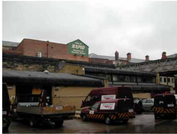
View of Back of Renshaw Street from site
