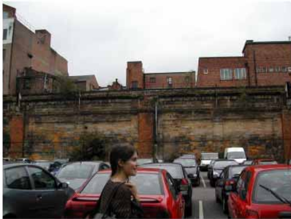
View towards Bold Street
