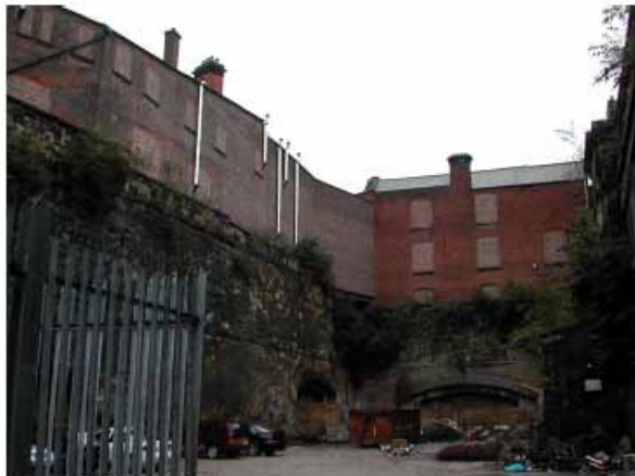
View of South East End of site
